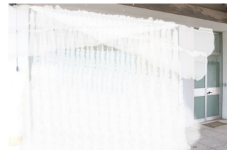
Barrier with water mist blade Spray-tecs installed in a compartment of access to industrial warehouse.
